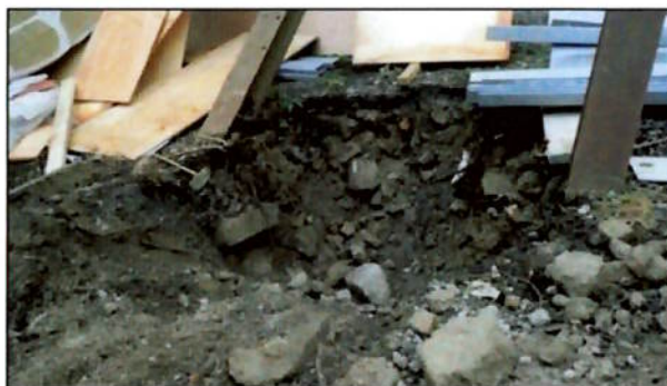
Figure 44 Trench 5, from the north
