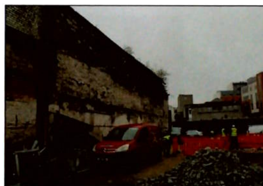
Figure 94 Building 4 from the east
