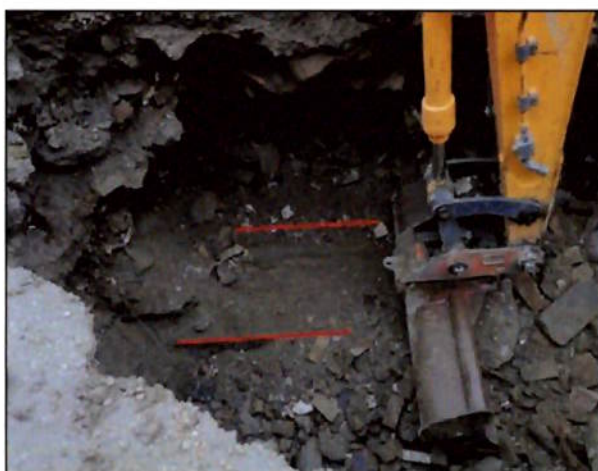
Figure 60 The structure from the north
