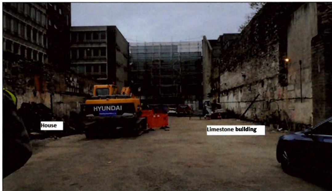
Figure 68 Site from the west
