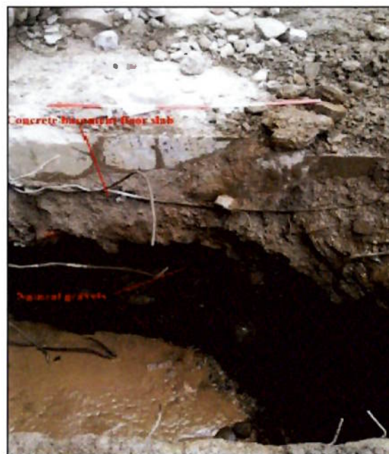
Figure 25 Trench B, concrete and natural gravels
