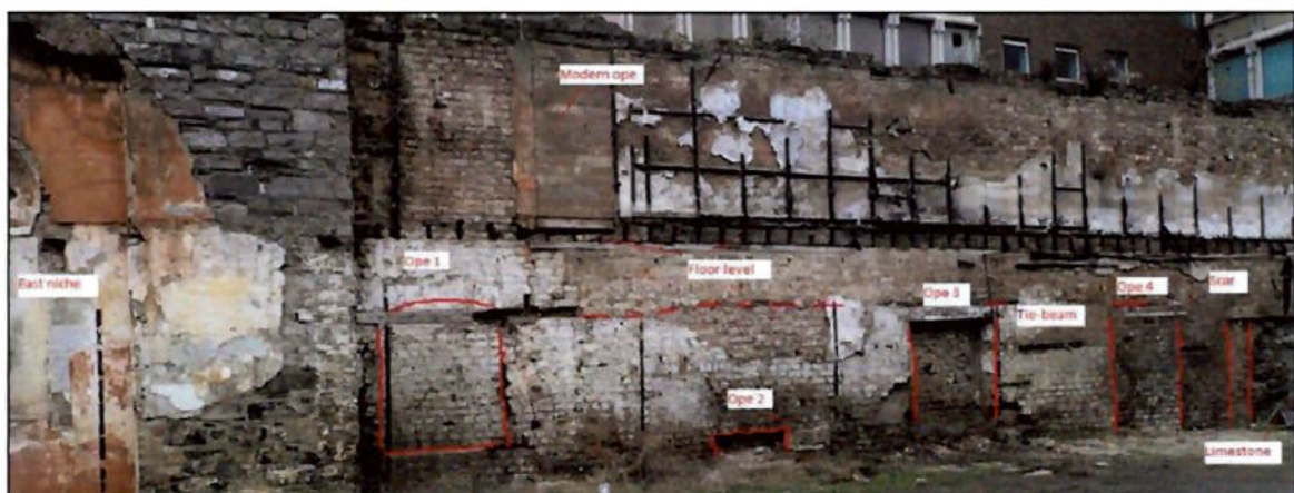
Figure 83 Building 3, from the west
