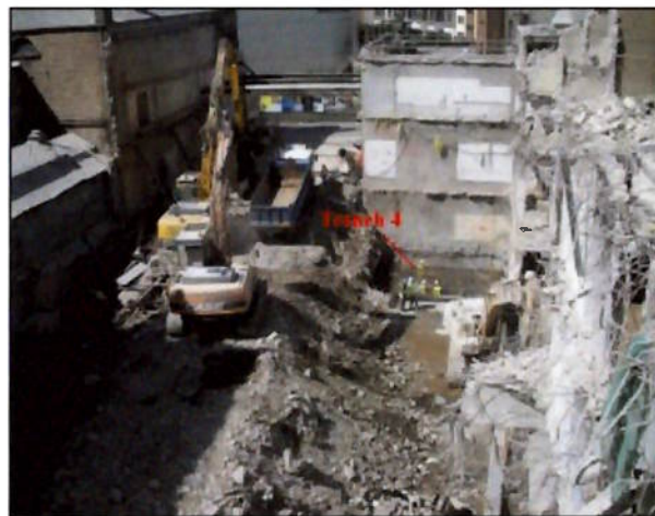
Figure 24 The site from the north, 2009
