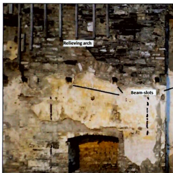
Figure 78 The relieving arch and beam-slots
