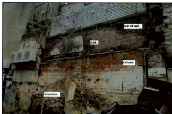
Figure 91 The boundary wall, at the eastern end
