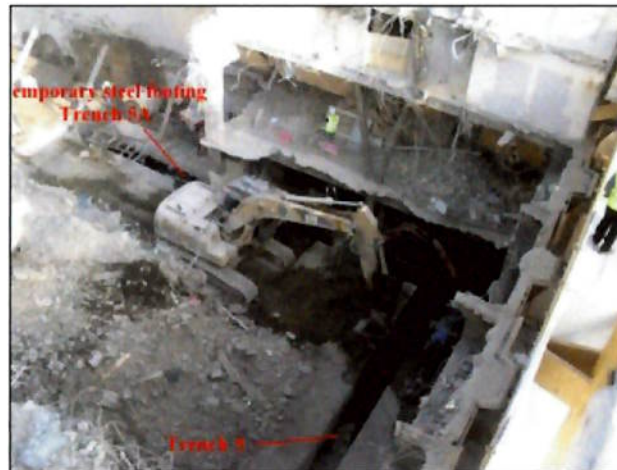
Figure 23 Overview of steel footing trench
