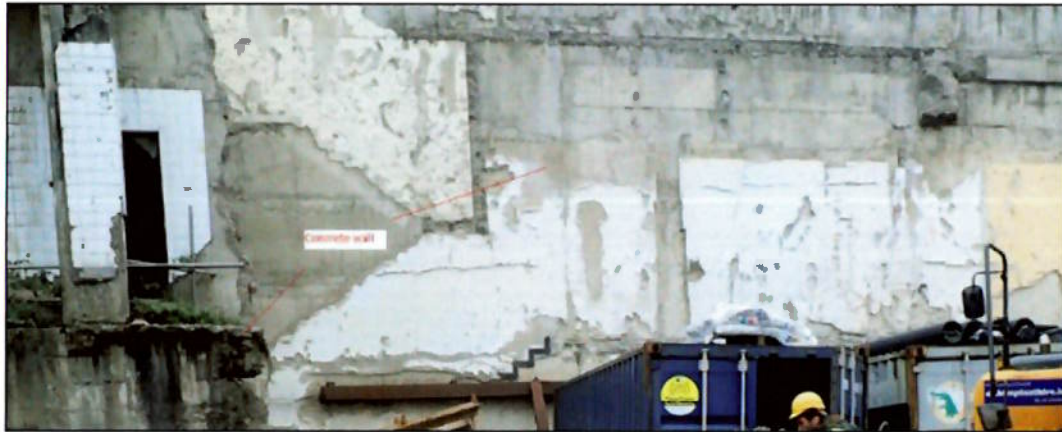
Figure 63 The north wall
