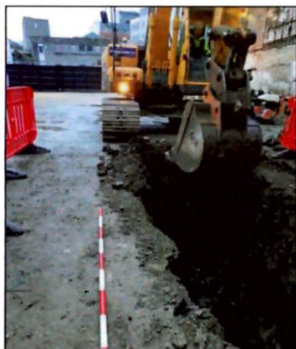
Figure 45 Trench 1, from the east
