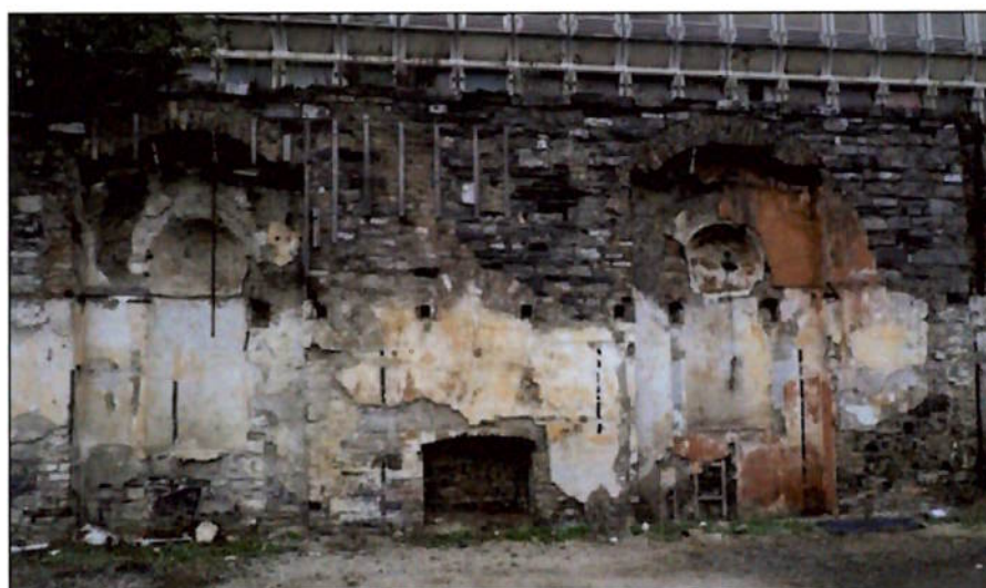
Figure 74 Building 2, from the south
