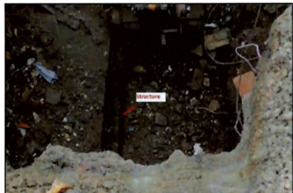
Figure 58 Foundation from the east
