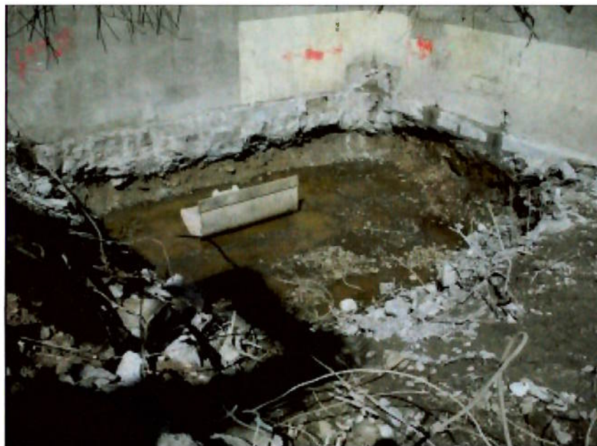
Figure 27 Trench 4, temporary crane base
